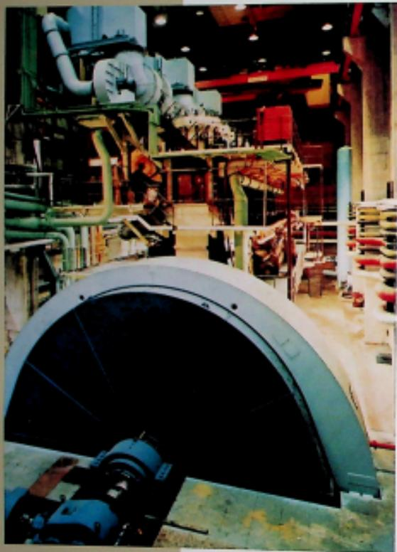
General view of a diesel generator set of 39.1 MVA equipped with a 40 000 H.P. two-stroke diesel engine.
